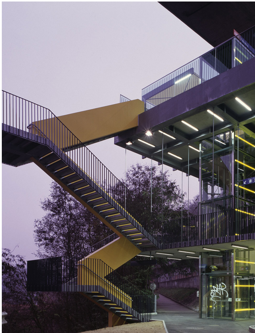
Neubau RBS Station Felsenau Bern Ebene Felsenau-Viadukt
